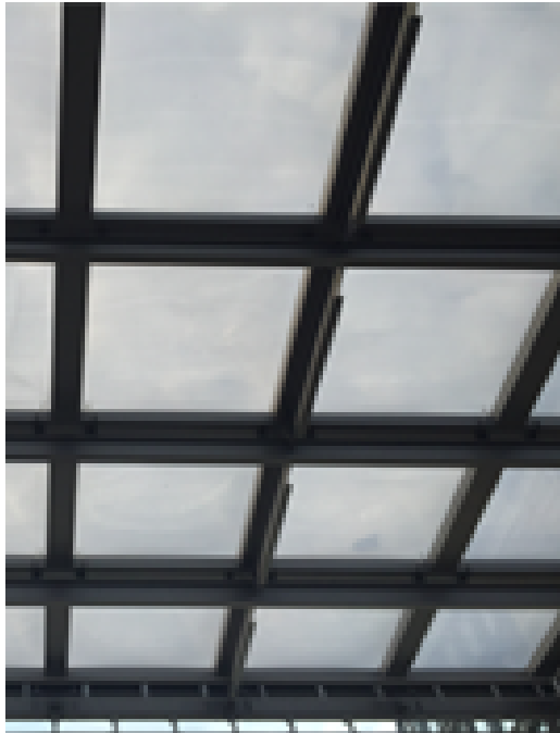
Cat A - real example of ETFE Roof
