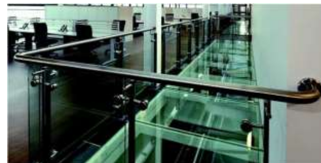
Cat A balustrade.
